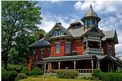
1093 Dwight Street Holyoke 1886 totally restored
